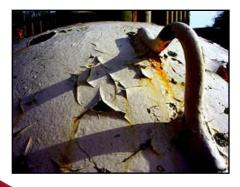
Tanks cannot be allowed to rust out and leak. White or silver paint is approved.
