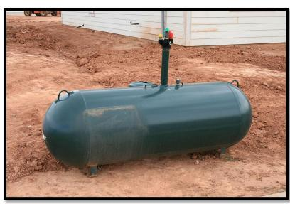
This LPG tank is coated and prepared for an underground installation.
